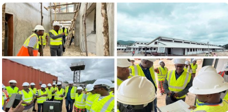
Office of the Minister of Health and Sanitation Monitors Infrastructural Development
