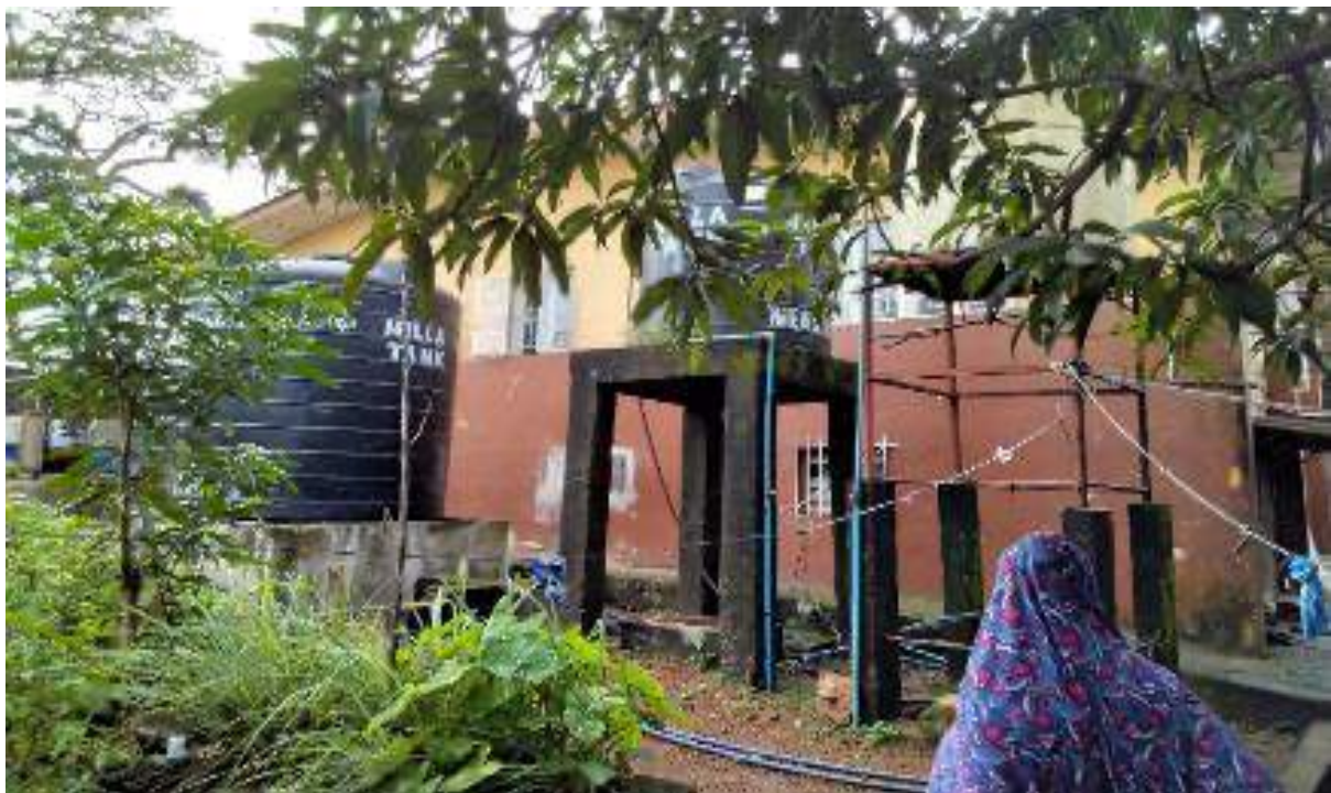
Plate 14: Existing Water Storage Tanks
