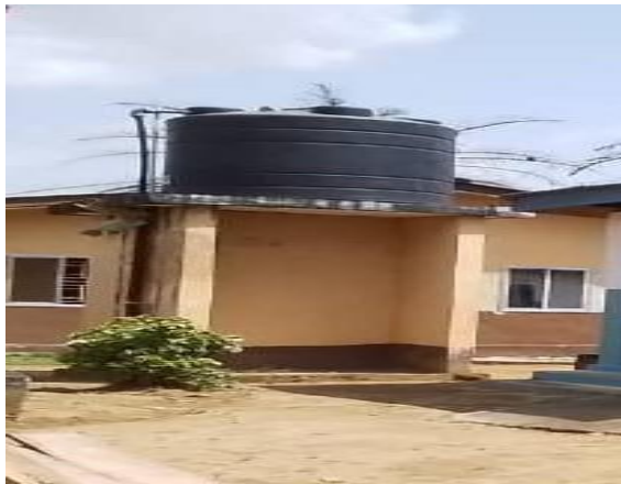
Plate 9: Elevated 5,000L Water Tank
